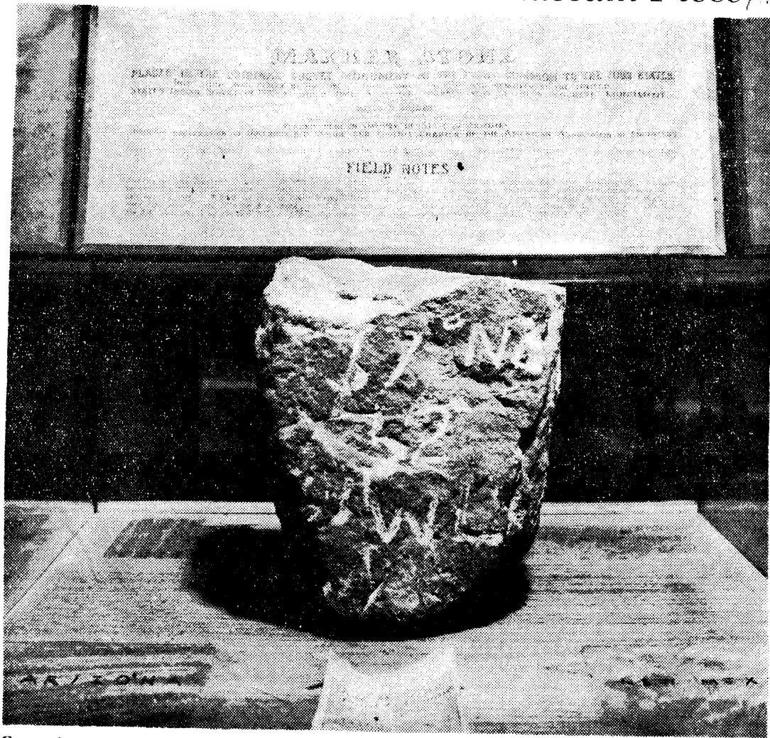
Cornerstones usually are found in buildings of size and distinction; but here is a "four corner" stone that was one of the most unusual markers in the United States. From 1875 until 1932 it lay at an inaccessible point that marked the joining of Colorado, New Mexico, Arizona, and Utah state lines. There is no other such geographical distinction in the nation. The surveyor's marks indicate 37 degrees, North Latitude; 32 degrees West Longitude from Washington. On top the date 1875, is cut. The stone now is exhibited at the state library museum.—(Republic Staff Photo)
