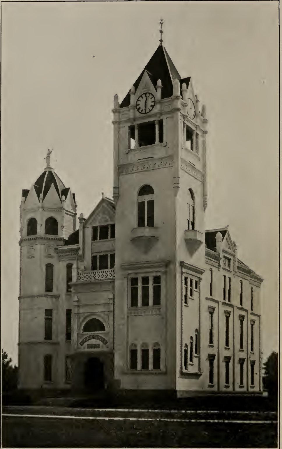
Linn County Courthouse at Albany, Oregon, where Puter and McKinley operated extensively through Deputy County Clerk Robt. B. Montague
