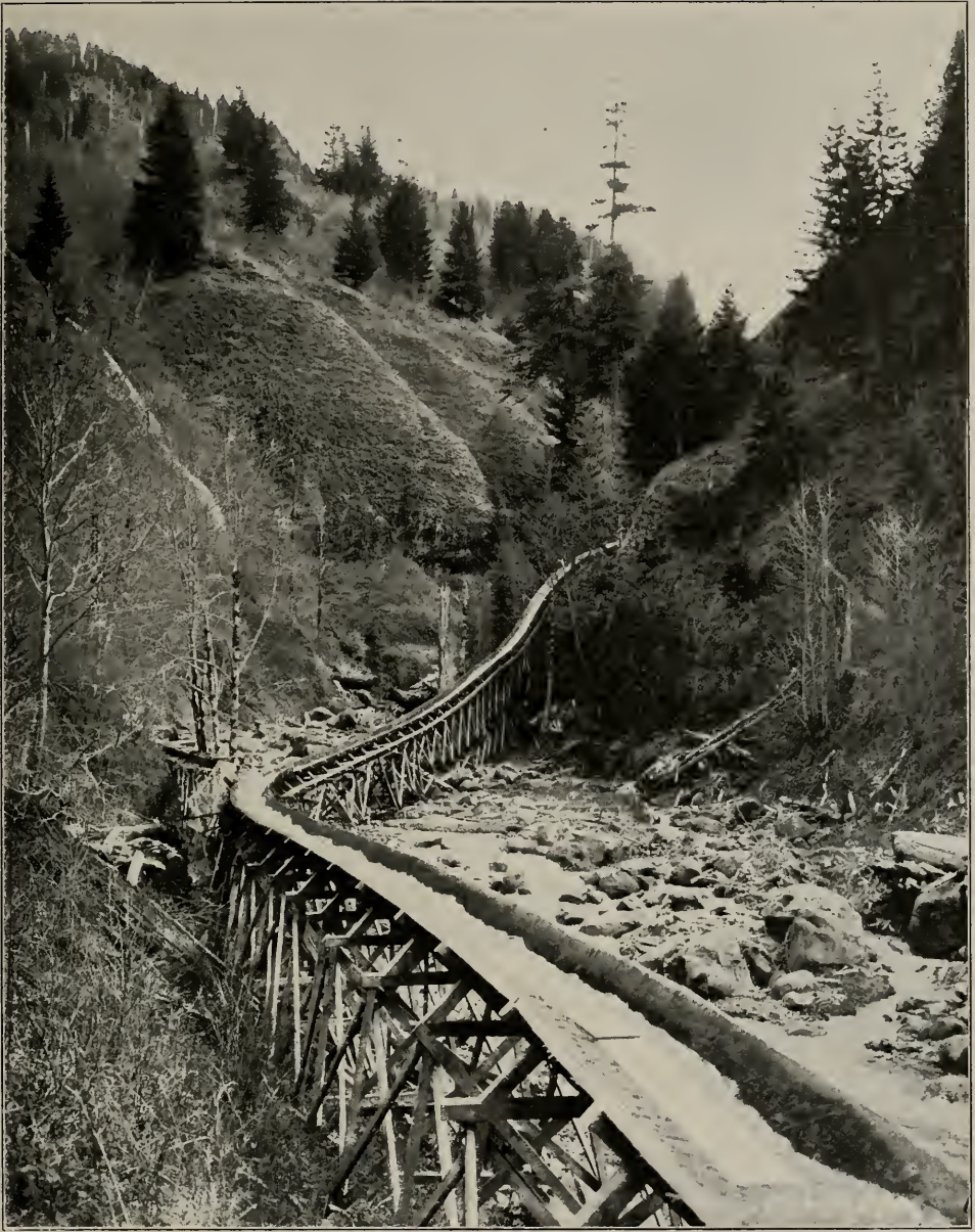
Lumber flume at Bridal Veil, Oregon, having a drop of 2,500 feet in two miles. Timbers 12x12 and 60 feet in length have come down this flume
