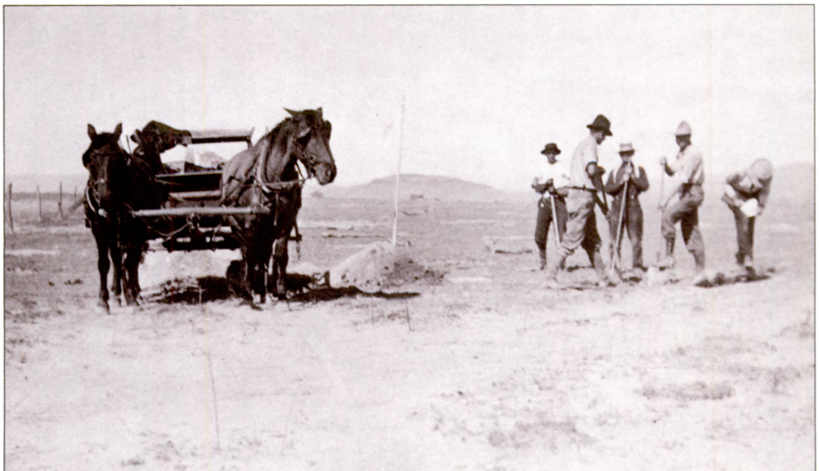
Survey crew setting a wooden corner stake.
