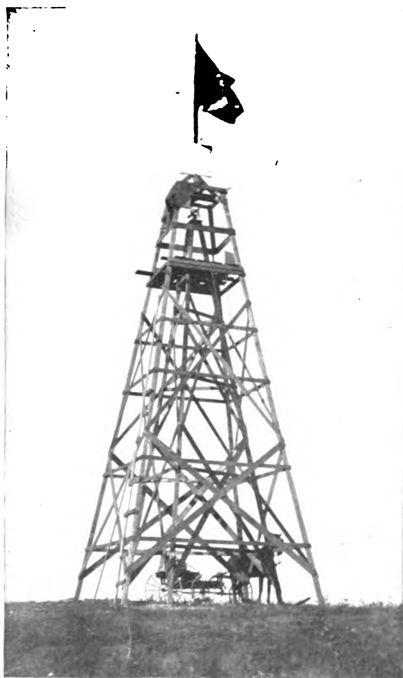
FIG. 165.—OBSERVING SCAFFOLD AND SIGNAL.
